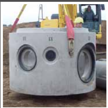
1500 mm diameter Sealed Manhole Base Unit
