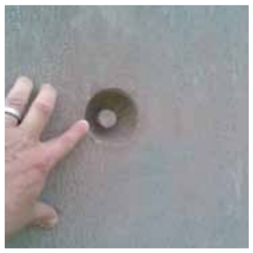
Photo showing 'cast in' DEHA anchor pin on the side of Manhole unit.
