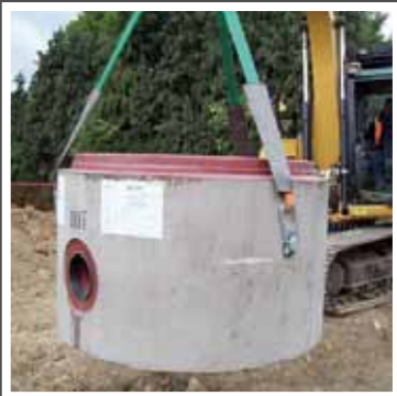
1200 mm diameter Sealed Manhole Base Unit
