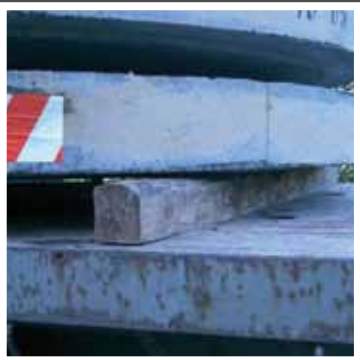
Image 1.0 / Large cover slabs are loaded with full length timbers in between each unit.
