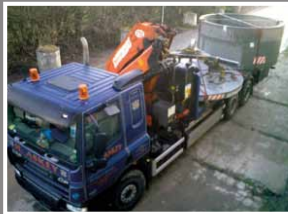
Six wheeler rigid with ‘Crane Off-Load’ behind the cab facility loaded with large manhole and cover slab units.
