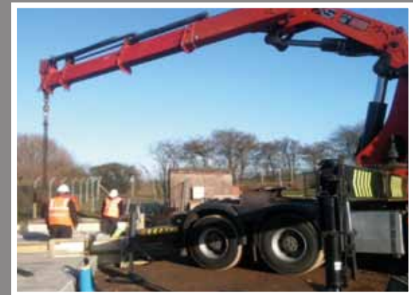
Crane mounted articulated unit with behind the cab crane. This vehicle is equipped with detachable trailer. The artic unit is then allowed to manoeuvre the product into position. This unit has a high capacity lift radius.
